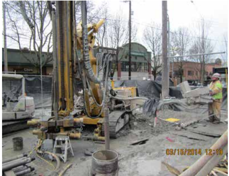
Testing underground conditions sometimes involves working in city-center locations.
